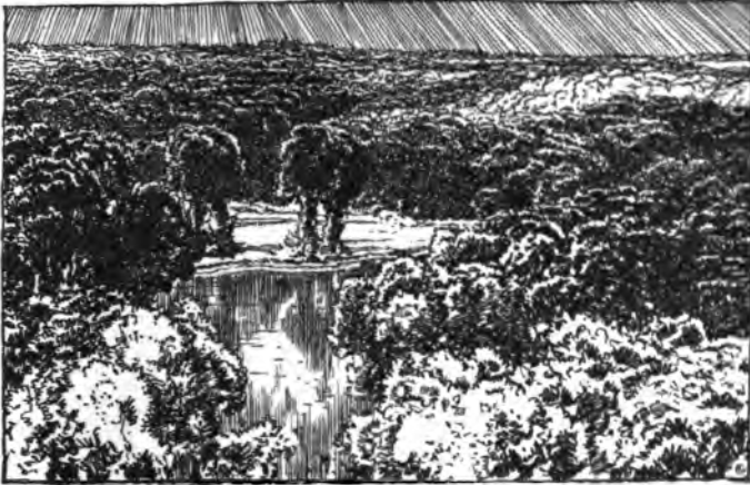
The Maran Valley from the Viaduct.
